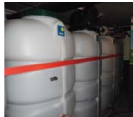
Figure 2: Lower reservoir and Pelton turbine of the Goudemand residence pumped storage hydro (in 2015).
